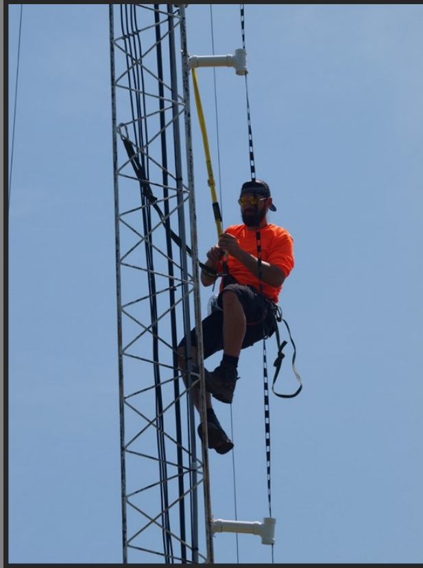
Matt securing himself and transmission lines
