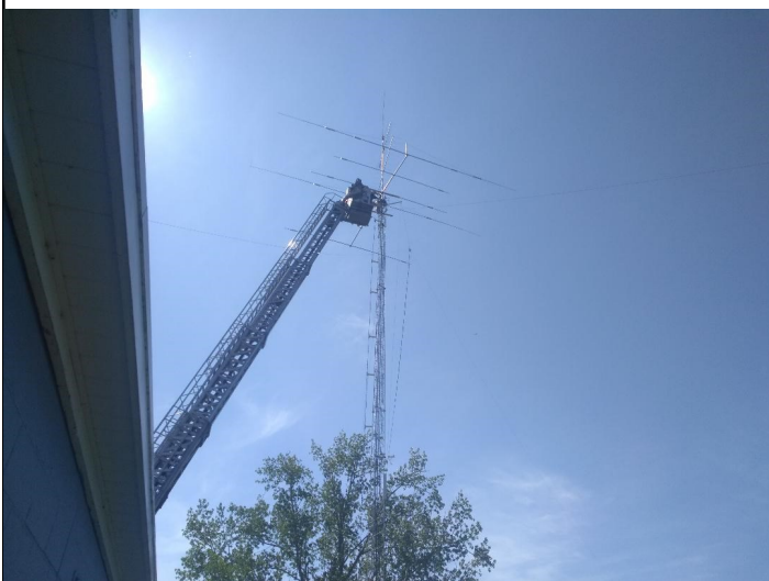
Tower ladder bucket working to secure mast to tower structure.
