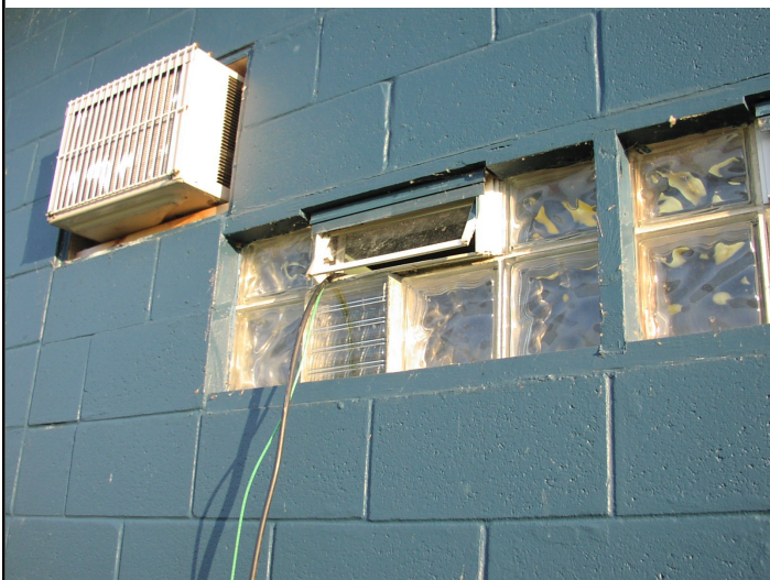
BELOW: GENERATOR FEED INTO RADIO SHACK
