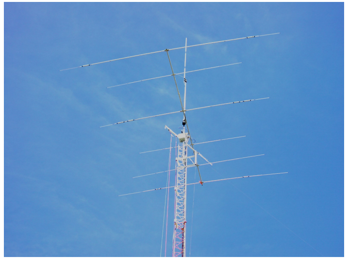
AFTER THE BEAM...
