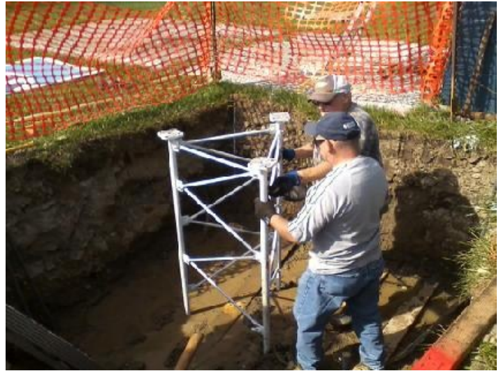
Above: Conrad Barrick and Ed Jablonski set the tower base.
