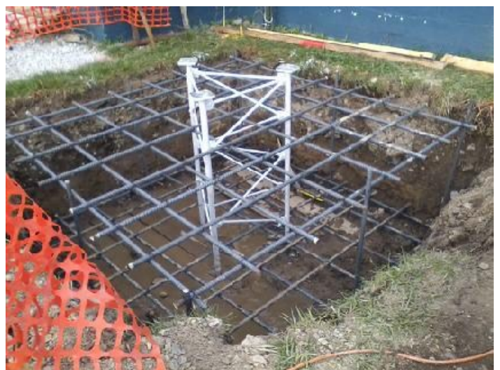
Below: Tower base and rebar cage complete and ready for inspection, form, concrete and tower installation.
