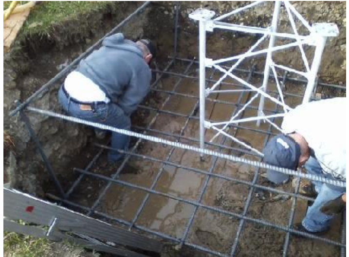
Below: Tower base and rebar cage complete and ready for inspection, form, concrete and tower installation.
